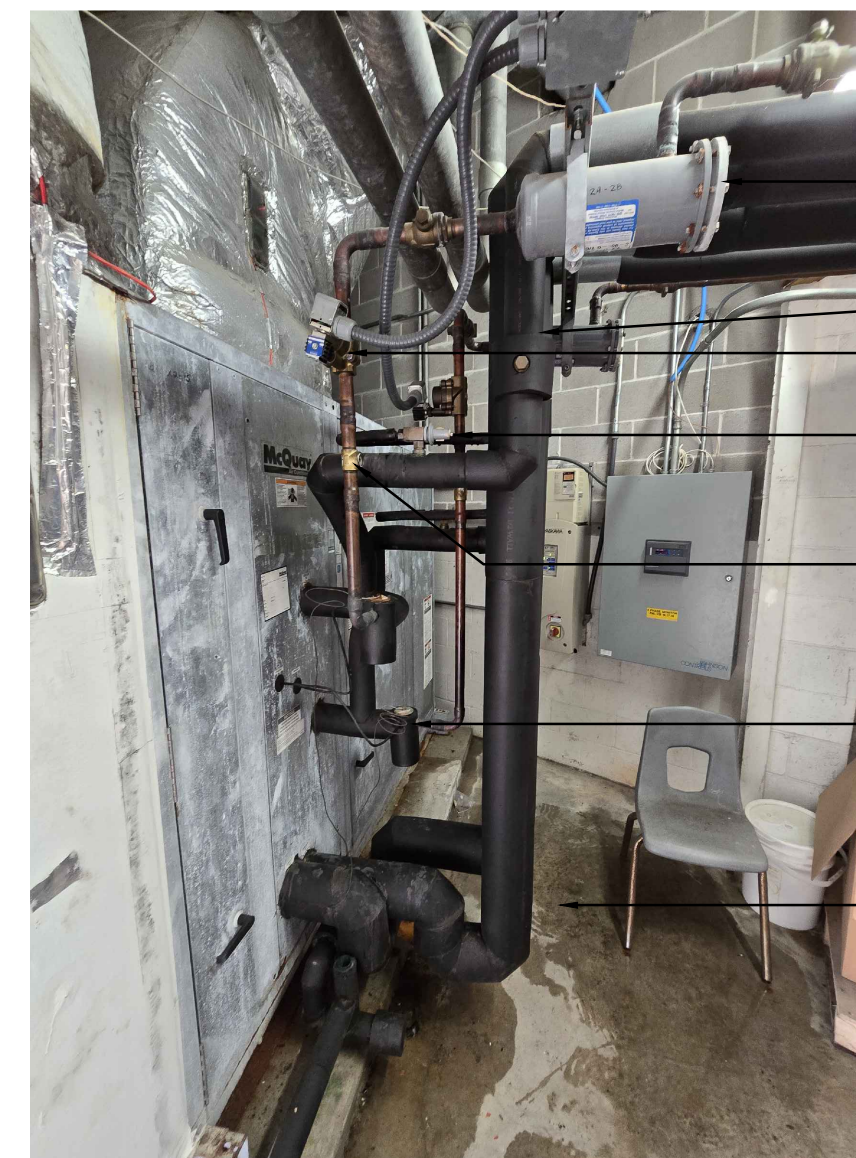
REPLACE EACH DRIER CORE WITH NEW INCLUDING GASKET WITH LEAK LOCK
